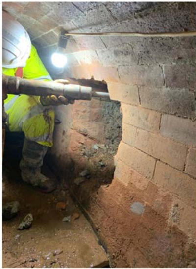
Devonshire Row Sewer – Repairing a collapsed connection
